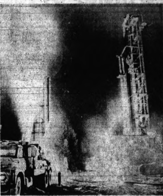
DRILLING CONTINUES — An engine drives a smaller drill (left) in the effort to open an access hole to three miners trapped since last Tuesday near Hazleton, Pa. The big drilling rig (right) began operation in the middle of the night.
