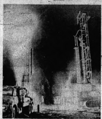
DRILLING CONTINUES — An engine drives a smaller drill (left) in the effort to open an access hole to three miners trapped since last Tuesday near Hazleton, Pa. The big drilling rig (right) began operation in the middle of the night.
