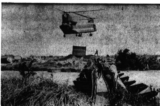
INSTANT CAMP — A Chinook helicopter sets a prefabricated bunker into a hole next to the Kinh Xang canal, about 15 miles west of Saigon where a semi-permanent camp was set up almost overnight. Troops of the U.S. 199th Light Infantry Brigade will use the bunker to defend the bridge.
