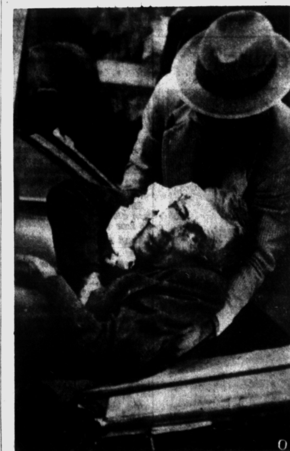
SOUTH LYON MAN INJURED — A South Lyon man and his wife were injured in Lebanon, Ohio, yesterday, when their car crashed into a loaded lumber truck at an intersection. Shown here, Donald Sayre, 72, of 60448 Nine Mile Rd., is being removed from the scene by ambulance attendants. The hospital they were taken to lists the conditions of Sayre and his wife as "serious."
