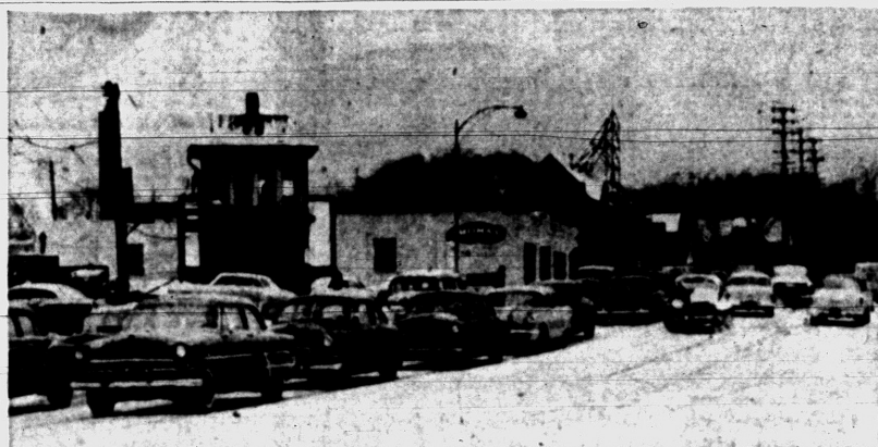
A TORTURED CRAWL—Mid-morning traffic in downtown Pontiac slows to a near-standstill as long lines of cars labor with spinning wheels over streets which have become glazed with an icy snow. The scene at the top was photographed along Wayne St. At the bottom, the cars on the right slid dangerously close to a column of almost-halted cars.
