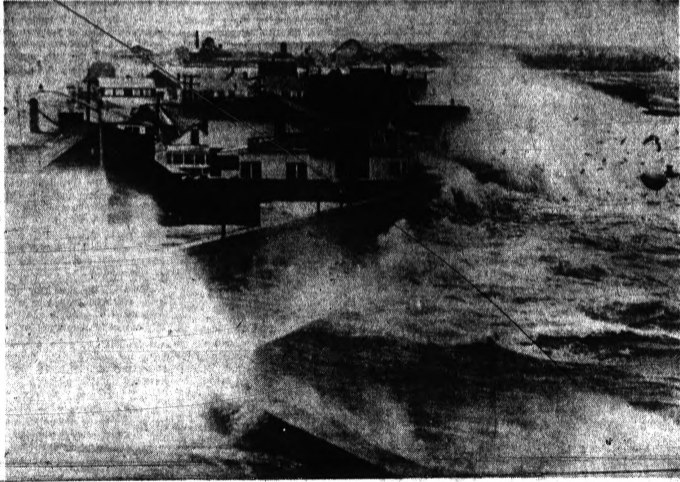
SURF BREAKS OVER SEAWALL —Waves break over the seawall at Winthrop, Mass., as gale winds batter the New England coastline. Some flooding occurred at low-lying areas. All along the coast, thousands fled their homes and damages are expected to run into the millions of dollars. Twenty deaths have been counted during this violent storm of late winter.
