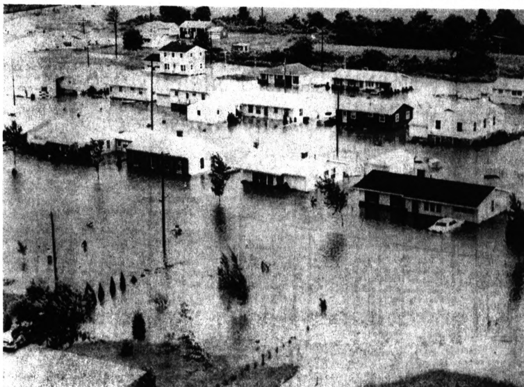
Low-Lying Areas Of Sandusky, Ohio, Flooded By Yesterday's Heavy Rains
