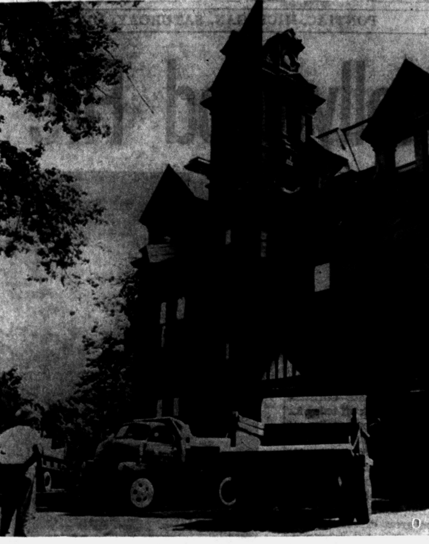
TREASURE TROVE?—Workmen dismantling the 30-room former lumber era mansion of Wellington R. Burt, richest man in Saginaw history, have orders to report any unusual "find" immediately. Some people believe the eccentric multi-millionaire may have secreted money or valuables somewhere between the walls of his cavernous east side showplace.
