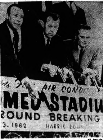
BREAK GROUND WITH 45 —The Houston Colts of the National Baseball League broke ground Wednesday in Houston for their multi-million dollar domed stadium due to be completed in 1963. Using 45 to break ground are (from left): Craig Culhnan, president of the club; Bill Elliott, Harris County judge; and Paul Richards, the club's general manager.
