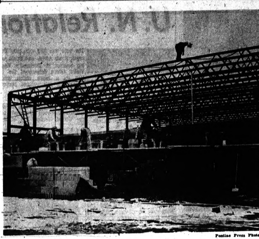
SCHOOL GOING UP — Construction is well under way on the new West Junior High School in Rochester being built on Old Perch Road between Avon Road and Walton Boulevard. The main section of the building will accommodate 600 students. Capacity will increase to 900 when a two-story wing is added later. Part of the current $1.1 million building and expansion program in the Rochester Community School District, the facility is slated to be ready for occupancy next September. Schurr Construction Co. of Pontiac is the general contractor.
