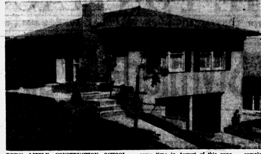
REDS' LITTLE CONSTRUCTION SCHOOL—Model home, above, at San Bruno, Calif., which Soviet building experts saw on their tour of the United States last fall, is prototype of one scheduled for shipment to Moscow
