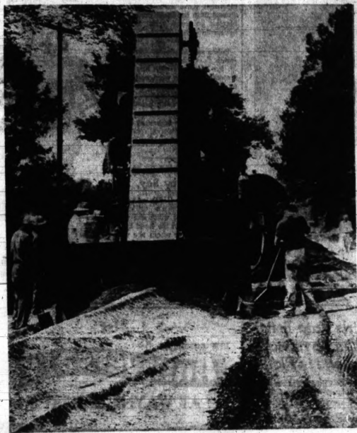
FIRST ROAD PROJECT —Wixom started its first road-paving project yesterday since becoming a city with the "stabilization" of Potter Road. The huge machine is an asphalt road plant and
