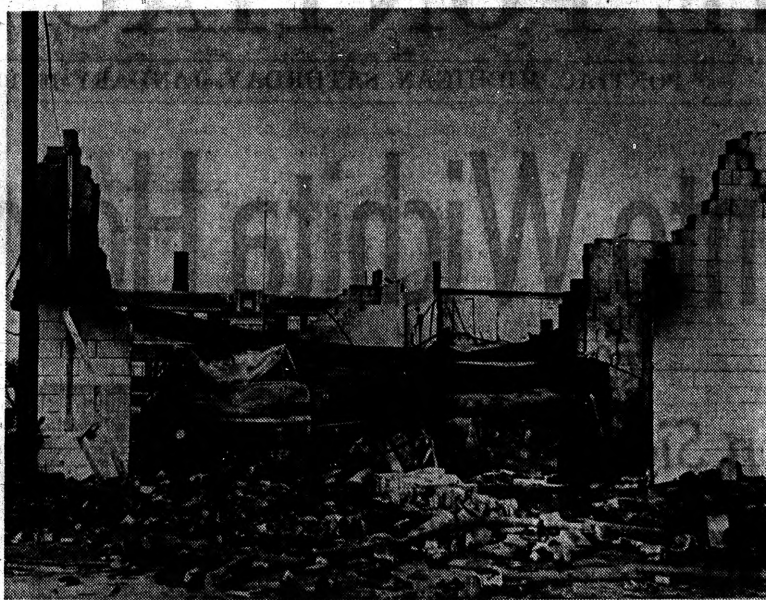
NINE-HOUR BLAZE —Pontiac firemen battled flames at this service station at 1430 Joslyn for more than nine hours last night and today. Hampered by a lack of water, high winds and near zero temperatures, fire
