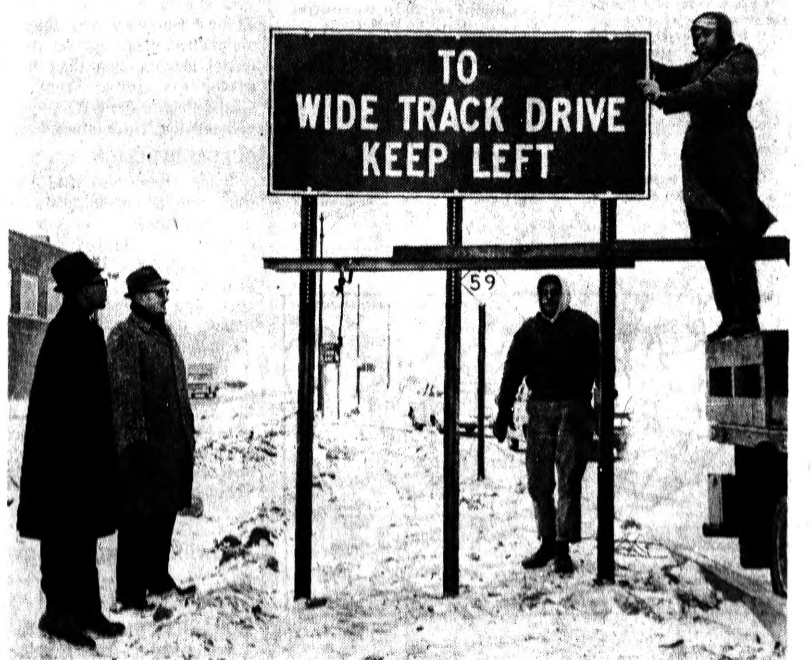
TO GUIDE MOTORISTS—Marcus Bradford (left), assistant district traffic engineer for the State Highway Department, and Joseph Koren, city traffic engineer, watch as a highway department crew installs a new direc-
