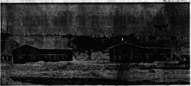
Apartments Rise On The Mill Pond Site
