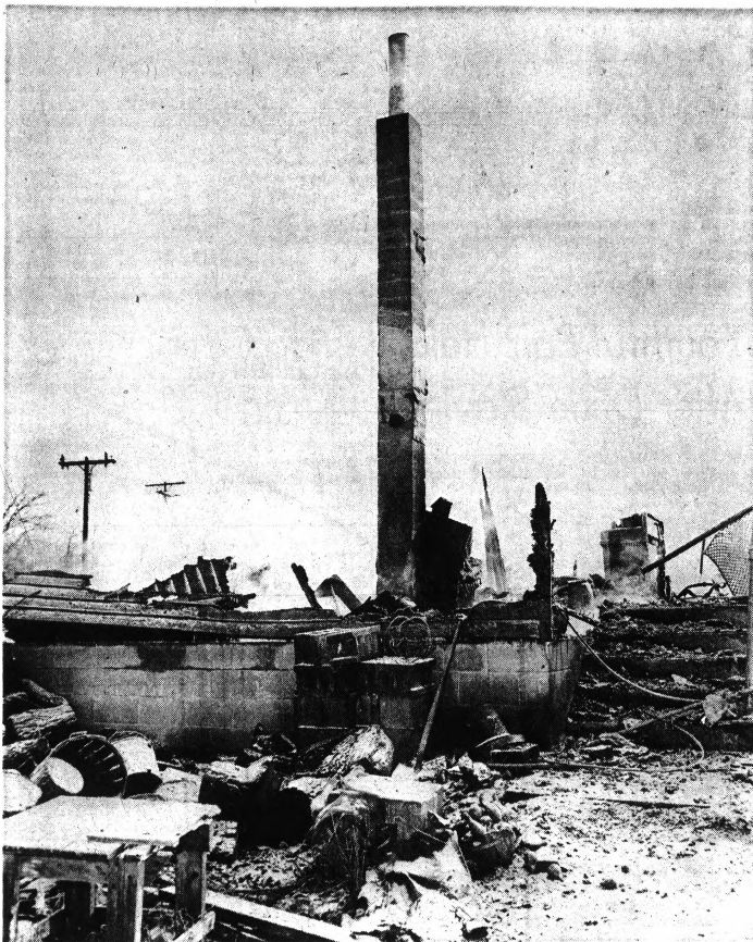
Remains Of White Lake Township Home Ravaged By Five-Hour Blaze
