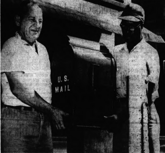
RELOCATION — This mailbox has been standing on the corner of Saginaw and West Huron Streets for more than 65 years, according to veteran postal employees. Lawrence Howard (left), engineering superintendent at the Pontiac Main Post Office, and a postal employee, Clifford A. Steele of 19 Elizabeth St., are shown removing the box. It has been replaced with a modern "snorkle" combination mailbox about 100 feet away because it blocked the vision of motorists.
