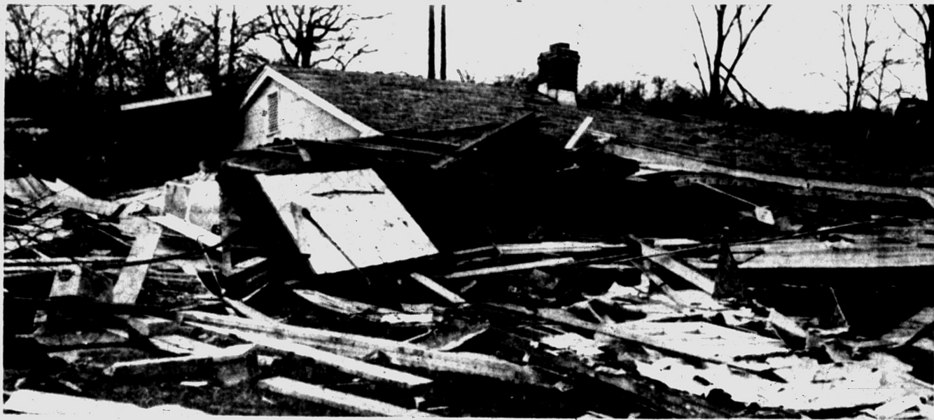
An Intact Roof Shelters the Rubble That Remains of This New Hudson Home.
