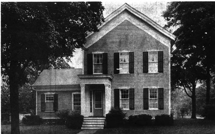
Dark Green Shutters Trim Painted Bronze Exterior Of The Fred Noyes' Home In Romeo
