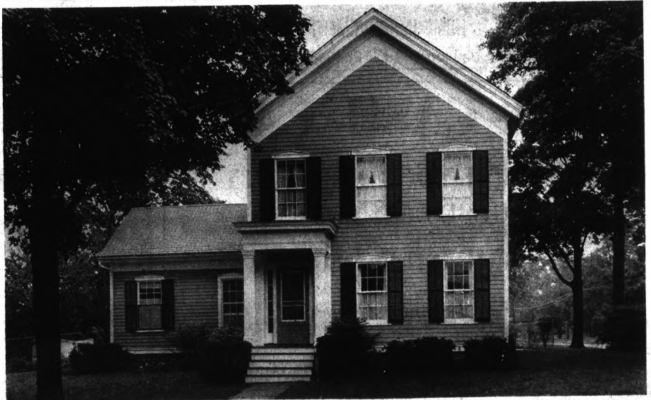
Dark Green Shutters Trim Painted Bronze Exterior Of The Fred Noyes' Home In Romeo
