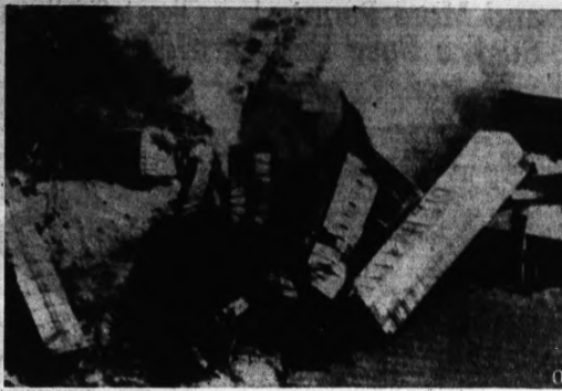
TRAIN WRECK —At least five people were killed and three injured when this Rock Island freight plunged off a flood-wrecked trestle 17 miles east of Tucumcari, N. M., Saturday. Seven
