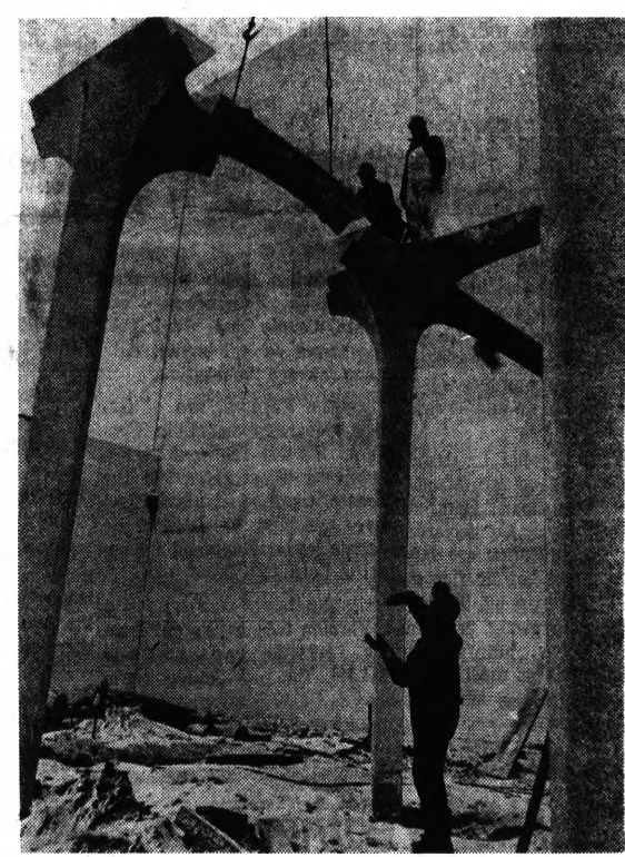
JIGSAW PUZZLE — Construction workers match pieces for a new entrance to the $2.4-million addition to Hudson's at the Pontiac Mall. The budget store should be relocated in the lower level by late February. The opening of a full-line store in the upper two levels is planned for late July.
