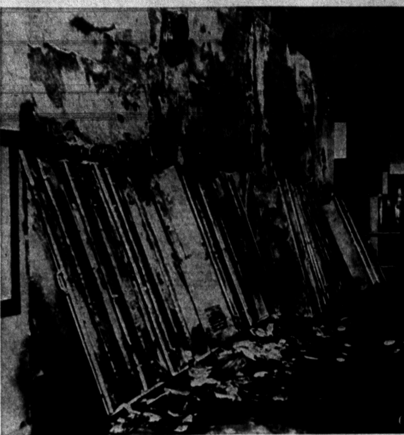
HIT BY FLAMES —A damage estimate of $200,000 has been placed on the fire which consumed portions of the Utica Junior High school early this morning. Some 500 pupils got an un-
