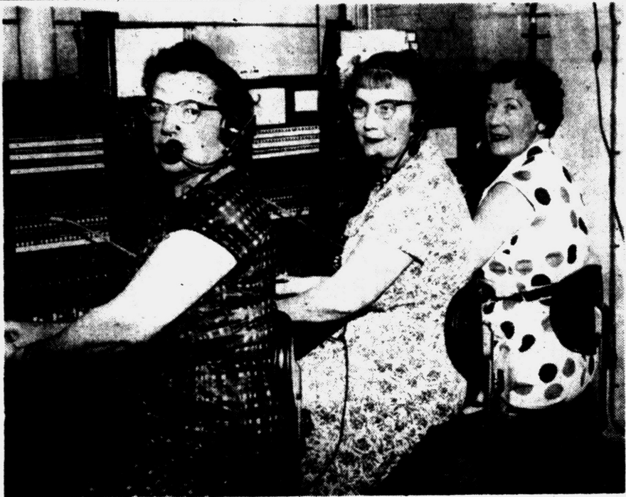
AT NEW COUNTY SWITCHBOARD — Oakland County's new and larger switchboard, located on the top floor of the County Office Building, was put into operation yesterday. It was installed to facilitate an influx of more calls to the county each day, which couldn't be handled by the old two boards. Operators are (from left) Mrs. Emma Rathbun, Mrs. Nettie Harrington, and Mrs. Genevieve Bale.
