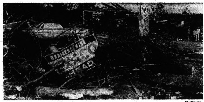
Wrecked Building, Twisted Trees Near Outing, Minn., Mark Tornado's Path
