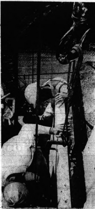
ANOTHER ONE IN PLACE — Workmen fit the heavy 4-by-4 marble slab in place after crane lowers it.
