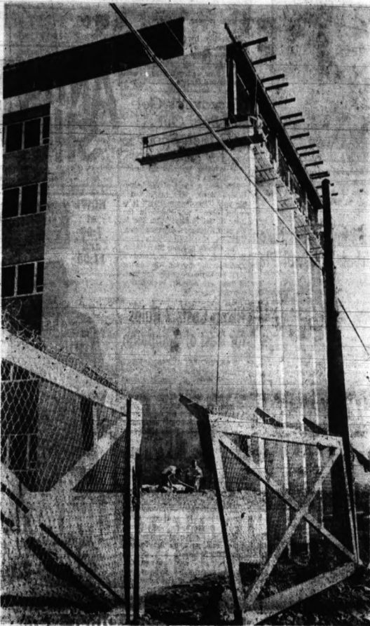
NORTHWEST CORNER — Workmen in the foreground demonstrate the size of Oakland County's new courthouse. The scaffolding near the top of the six-story structure is for the workmen adding slab after slab of the white Georgia marble facing.
