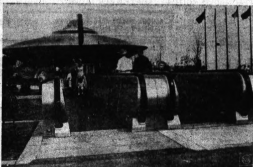
STEP SAVER — This is not a flat escalator. It is a moving sidewalk, something cities have used for years. This Speedwalk passenger conveyor system is installed in Freedland, a new amusement park in Bronx, N. Y.
