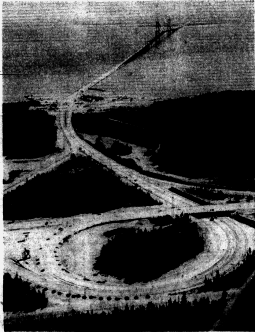
ST. IGNACE APPROACH — An aerial view of the north approach to the Straits of Mackinac Bridge shows the expressway-type system which connects the span to U. S. 2, west of St. Ignace. Ceremonies opened the bridge, linking Michigan's lower and upper peninsulas by land for the first time, about noon today. Cost of the northern approach was $1,357,000. The southern approach at Mackinac City, costing $1,429,000, offers connections with U. S. 23-27 and U. S. 31.
