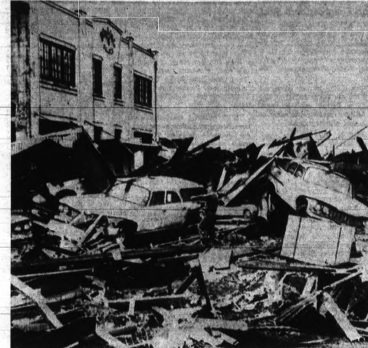
HILO SMASHED BY TIDAL WAVES — Automobiles tossed about like matchsticks amid the debris of broken buildings indicate the fury of four tidal waves that hit Hilo, Hawaii, early Monday morning. The waves, generated by earthquakes in Chile 6,800 miles away, took at least 33 lives, injured scores of others and damaged property to the extent of millions of dollars in Hilo alone.
