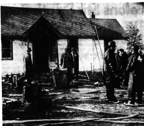
FIRE'S AFTERMATH — Firemen begin their cleanup after fire gutted this home at 4346 Forbush in West Bloomfield Township. The belongings of the Melvin Huntley family were destroyed in the blaze, from which three children narrowly escaped injury.
