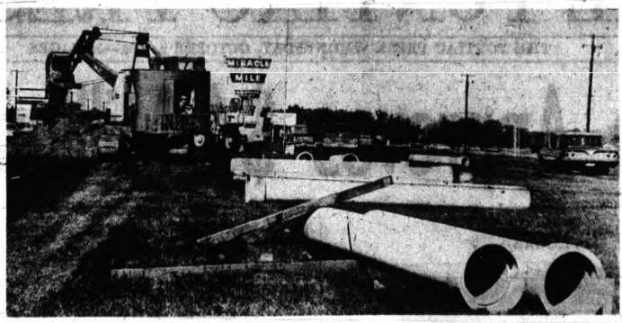
NEW WATER SOURCE — Construction of a $2.12-million pipeline to bring Detroit water to Bloomfield Township resident began yesterday. Digging of a 23-mile-long ditch started near
