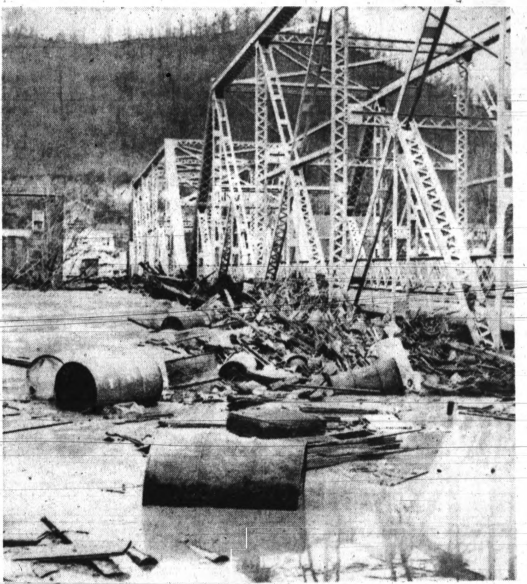
Flood Rubble Piles Into Cumberland River (Ky.) Bridge
