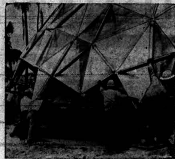
DIAMOND DOME —Something unique in construction is this aluminum-domed auditorium, shown during final stages of its erection at Honolulu's Hawaiian Village. Designed by Kaiser Aluminum of Oakland, Calif., the building was erected in only 20 working hours by a 38-man crew. There is no interior framework or support. Diamond-shaped aluminum panels are bolted together to form a rigid shell, which, as seen in lower photo, is strengthened by addition of exterior struts. The auditorium will seat more than 1,800 people.
