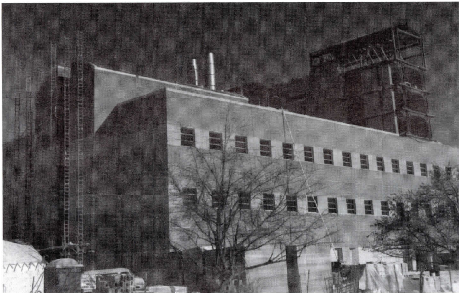
The new Science and Engineering complex, under construction.
