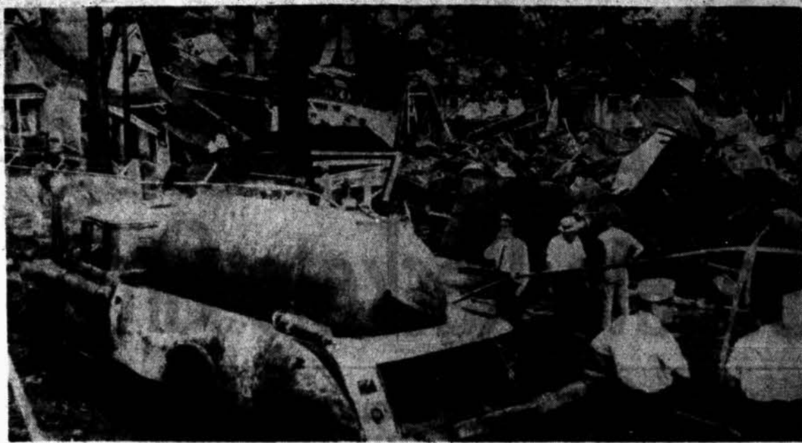
BLAST WRECKS AUGUSTA HOMES — Truck in foreground above is reported to be source of an explosion and fire which destroyed four homes in Augusta, Ga., Wednesday afternoon. The vehicle carried propane gas which is believed to have leaked through one of the hoses of the truck, causing the blast.
