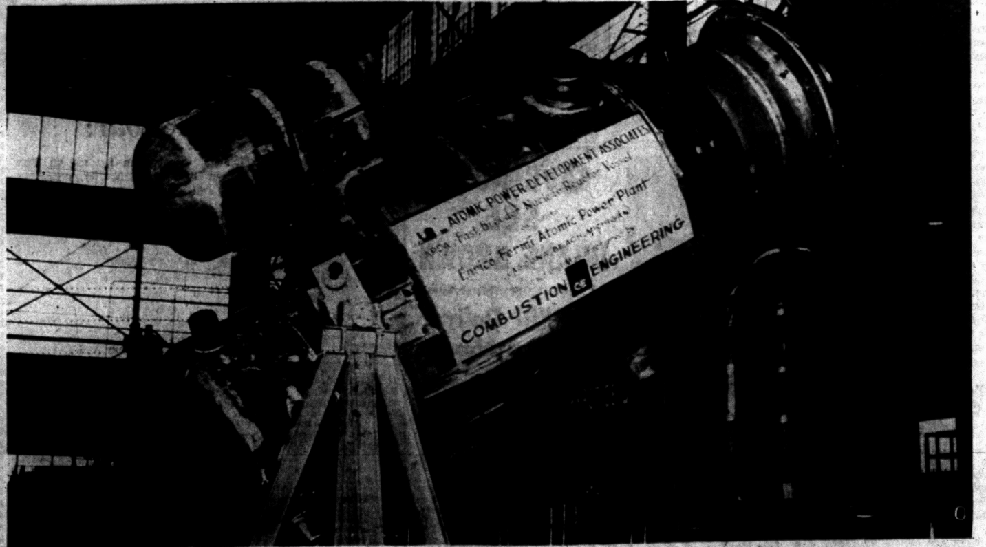
GIANT ATOMIC REACTOR — This is the 91-ton steel container — heart of the breeder reactor atomic power plant — now on the final lap of a 1,598-mile journey by barge and rail from Chattanooga, Tenn., to its ultimate site of operation, the Enrico Fermi Power Plant, at Monroe, Mich. The cumbersome cargo has created acute transportation problems during the long journey. The Fermi
