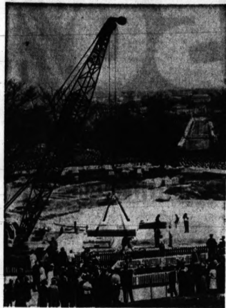
KENNEDY GRAVE SITE — A crane lowers a granite slab into place at the permanent site for the grave of President John F. Kennedy in Arlington National Cemetery yesterday. It was the first stone placed after its arrival from a quarry in Maine. In the foreground, visitors view the temporary grave of the assassinated president.
