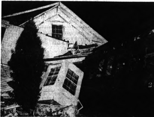
AN UNSCHEDULED STOP — Passenger car of an Erie Lackawanna train lies amid rubble of a house it hit at Peapack-Gladstone, N.J. The two-car train ran through a track-end
