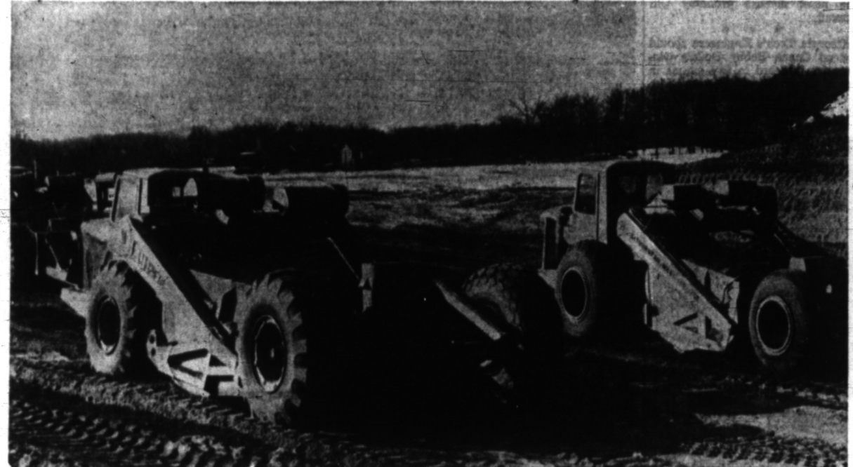
BIG JOB BEGINS —Heavy machinery for moving large quantities of earth are at work on the skeet range at Oakland County Sportsmen's Club, preparing for expansion of the range. The additions to be made will provide adequate facilities for the 1954 National Skeet Championships, to be held here.
