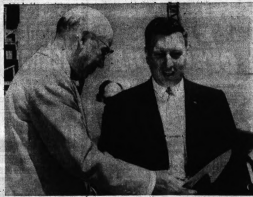
YOUR TURN — Last, but not least, to apply some cement to the base of the cornerstone was John B. Osgood (right), chairman of the Special County Building Committee which has been instrumental in the development of the new $3,000,000 courthouse. Handling Osgood the chrome-plated trowel is Luther Heacock, chairman of the Buildings and Grounds Committee of the Board of Supervisors.
