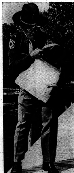
LIFE PRESERVER — Lt. Donald Kratt demonstrates the proper method of using a buoyant cushion as a safety device. One leg is placed through a loop of the Coast Guard approved cushion while the opposite arm is put through the other loop. Cushions should be checked periodically as they lose buoyancy through constant use as seats.
