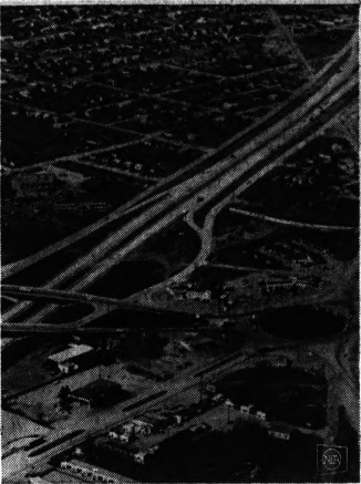
HIGHWAY RIBBONS —Laid through the suburbs of Waco, Tex., are ribbons of superhighways dividing the homes on the left from those on the right. Home owners will fall asleep each night to a lullaby of singing rubber on concrete.
