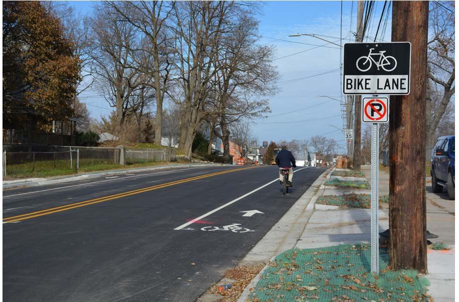
Construction crews recently put the finishing touches on Saginaw Street, north of the downtown, to define on-street bike lanes in Pontiac.
